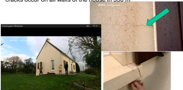
Figure 1: Cracks in a house occur in a distance of app. 350 m to wind turbines [1].
